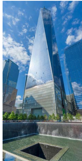
The Freedom Tower and one of its Reflecting Pools.
